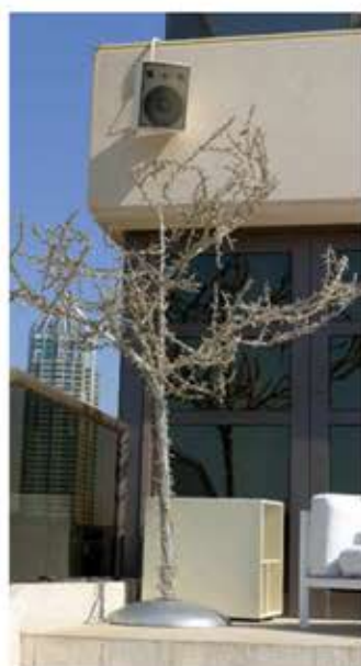
Cabling was the biggest challenge at the Grosvenor House Hotel
