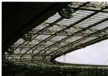
Paris-based manufacturer Nexo has continued its association with the Stade de France by designing a system around its new Geo array for the arena's 'Village' retail spaces
